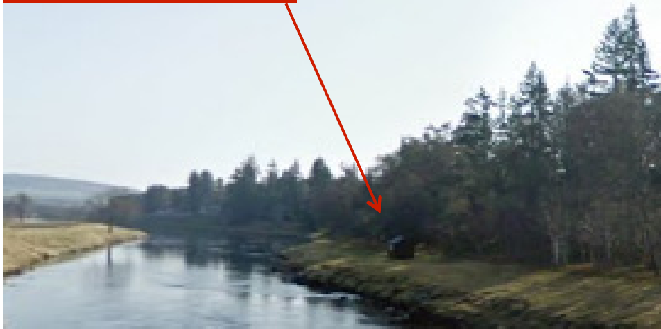
View of existing fishing hut from Dinnet Bridge
